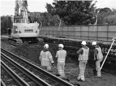
Heading south, the second project is the replacement of an under bridge (no.255) just north of Long Martin station. This involved the fabrication off site of a new concrete deck weighing 86 tonnes. This was manoeuvred by a hydraulic lift vehicle and lowered onto the two original side walls, which had been cut back to accept the new structure. The new bridge is not very pretty, but it is robust.
