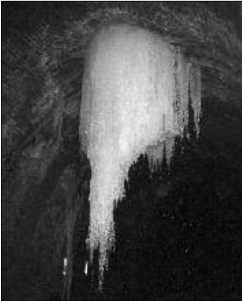
An icicle which formed inside Blea Moor tunnel during the 'big freeze'.
