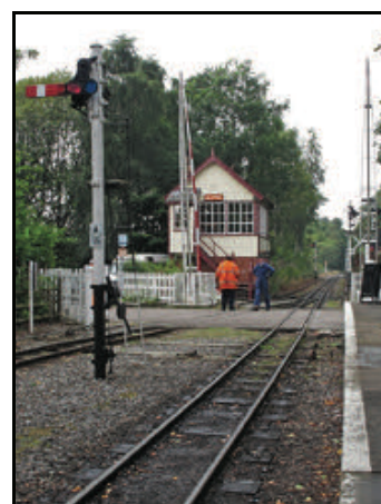
6: Starter signal, crossing & signal box at Alston Local efforts to preserve the standard gauge line were unsuccessful and BR removed the track. Narrow gauge trains now run on approximately 2½ miles of two-foot gauge track laid by volunteers along the old trackbed between Alston & Kirkhaugh. Photograph by Mark Harvey
